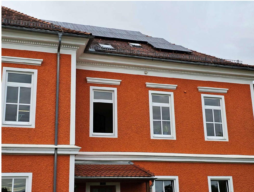
PVA - Dach Kindergarten Nord-West (20,25 kWP)
